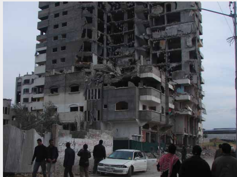
Al-Andalus apartment building which was bombarded by Israeli warplanes
